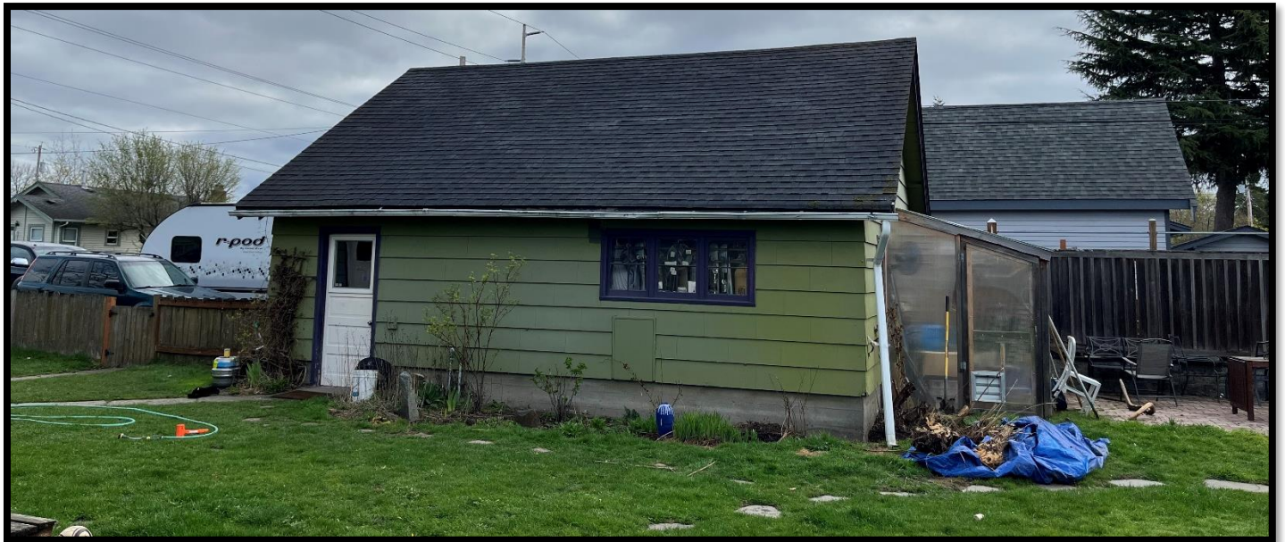
Image 2: Project site conditions at 2530 Jaeger Street with the existing garage in center. Facing east on March 26, 2024.
